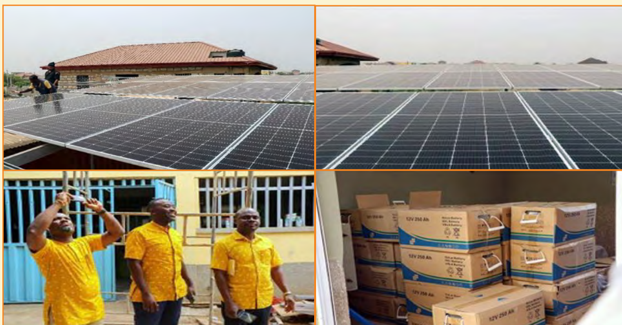
Installation of 150KW Solar PV System for Satchet Water Production
