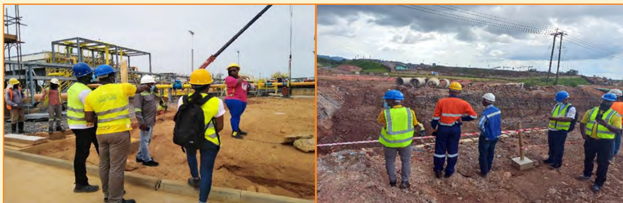
Monitoring visit to ensure adequacy of implementation of ESG management measures
