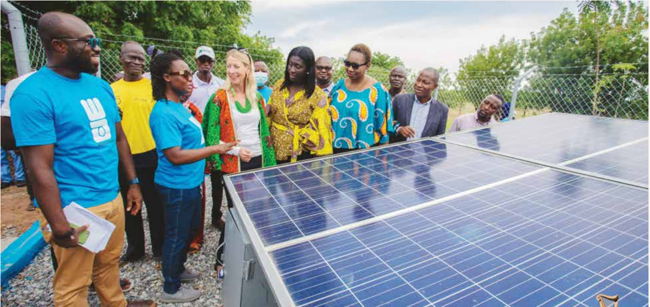
WASH Project at Sabuli in the Jirapa district (Upper West region) is solar powered
